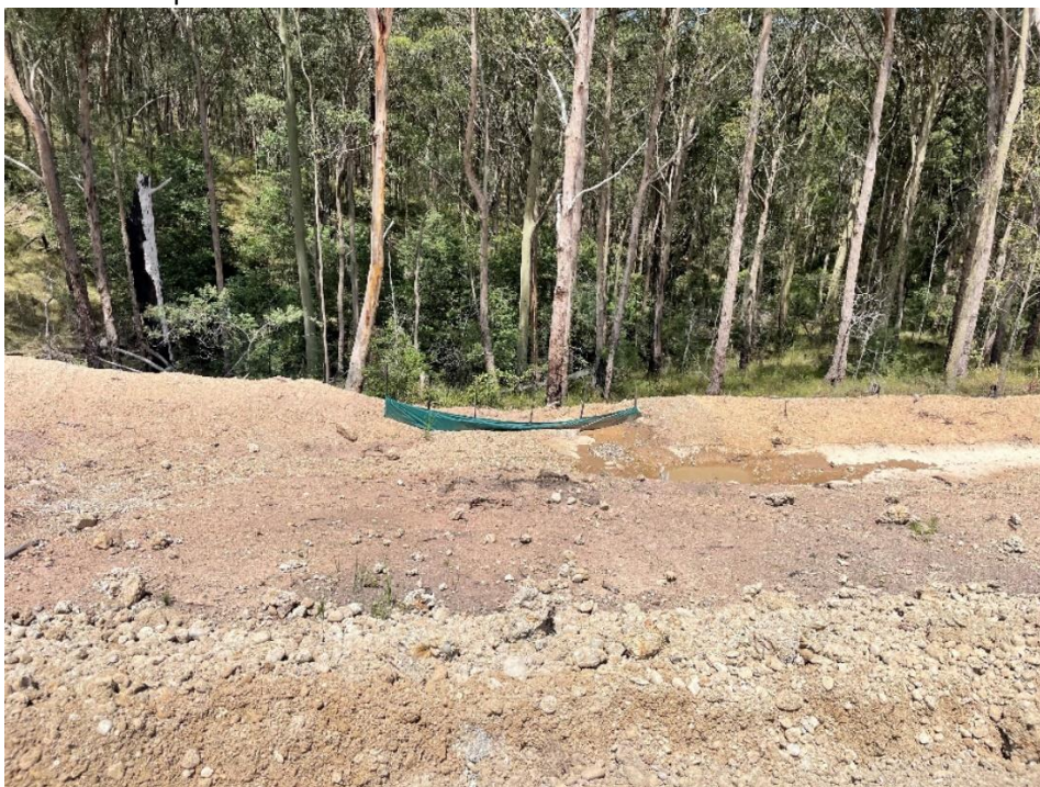
Sediment fence at surface water outlet.
