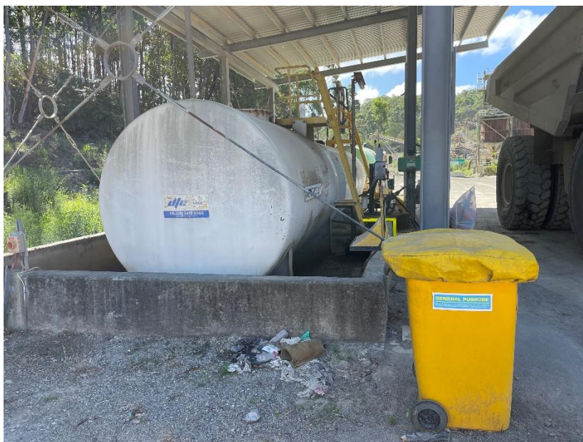
Above ground storage tank with spill kit nearby
