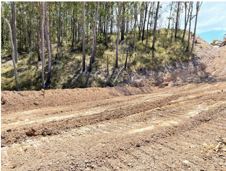
Gravel berm provided for erosion and sediment control
