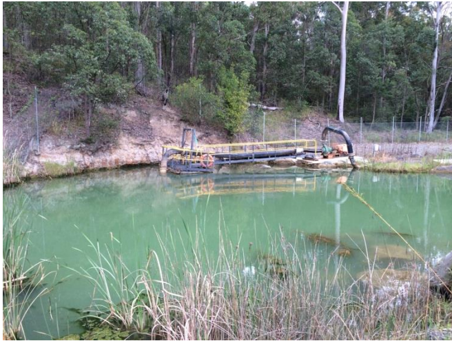
Plate 7.1 Mine Adit Dam
