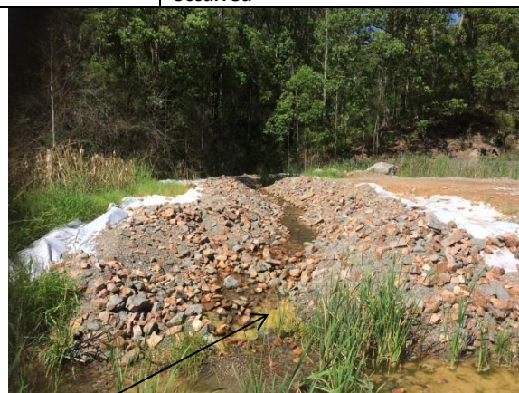
Water discharge from Dam A (Mine Adit Dam) following 100mm rain 2-3 March 2014 was compliant with the EPL discharge criteria.
