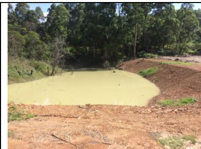
Runoff water collected in Dam D following 100mm of rain on 2-3 March 2014. No discharge to Dam C or Dam B downstream occurred
