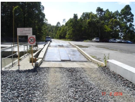
Wheel wash – exit to Railway Street from Southern Extraction Area
