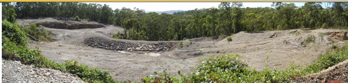
Dam K – eastern Mid-Pit (capacity 2ML) north of Rhondda Road. Total capacity still available after the February or March 2014 rain events.
