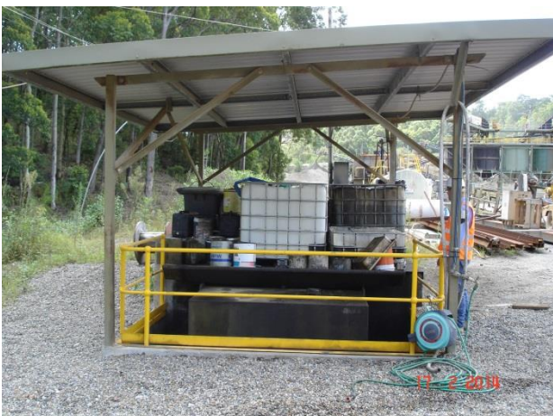
Waste oil bunded storage area adjacent to the on-site workshop.
