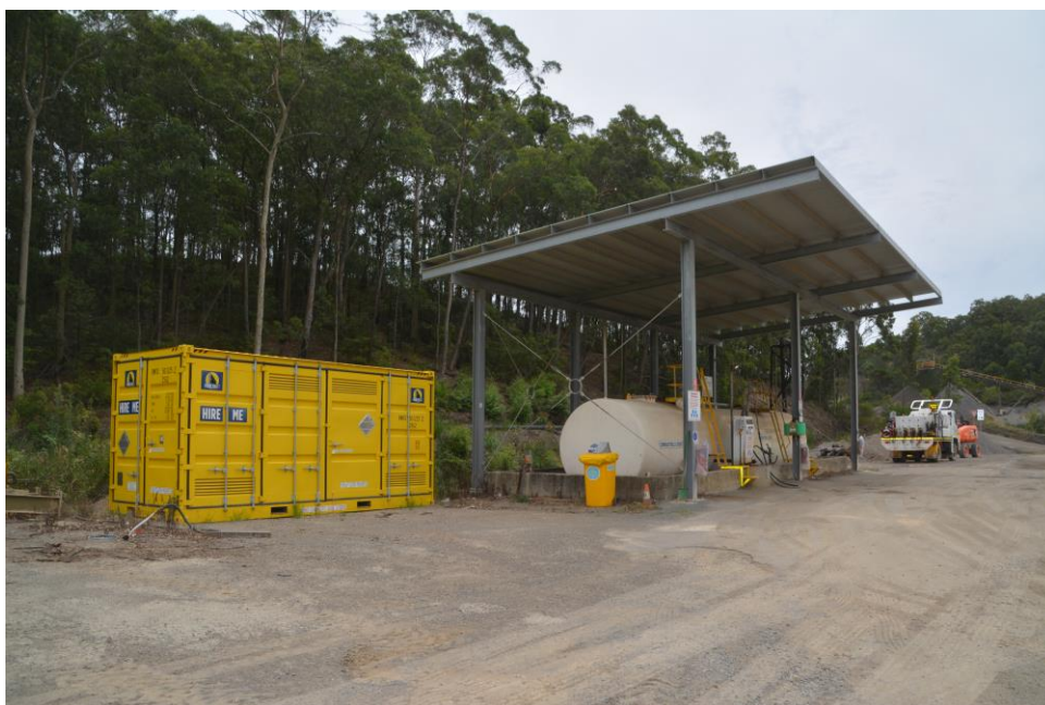
Plate 10 Portable Oil Storage Container (Ref: E559AH_143)
