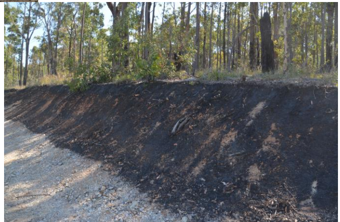
Plate 8 A view of the bitumen treatment of the upper extraction bench in Stage 1B (E559AG_055)
