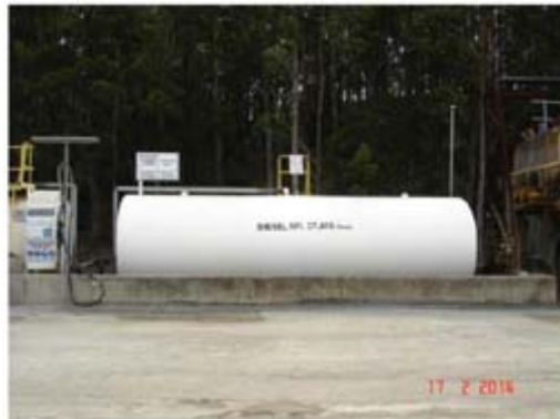
Bunded diesel tank adjacent to the waste oil and grease storage area.
