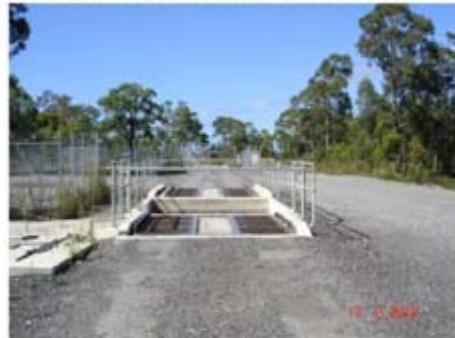
Wheel wash–exit to Rhondda Road from the Northern/Mid-Pit Area.
