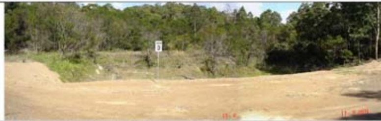
Dam D - Vegetated sediment dam with the dam wall to be raised 2m to increase the capacity to 25ML. Total capacity still available for collection of runoff water after the February 2014 rain event.
